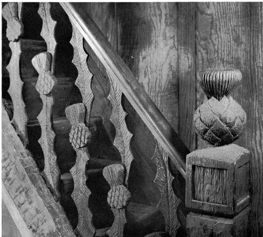
A section of the rugged and handsome stairway to the Croft loft guest quarters of Mrs. Agnes MacRae Morton's home. Newel post and stair-rail were designed and hand-carved in thistle motif by son Julian.
